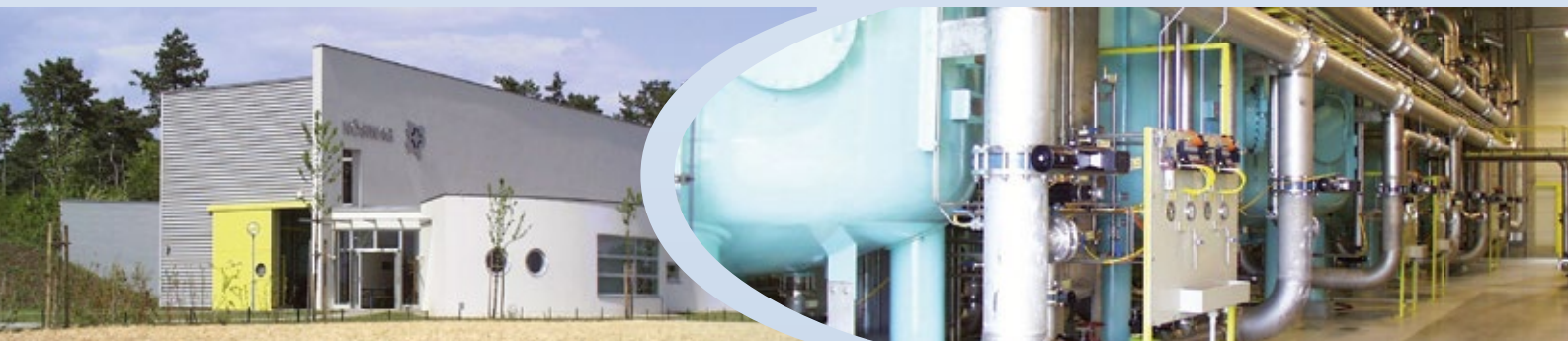
Obersiebenbrunn, Austria Commissioning 1997, 4'320 m 3 /d
