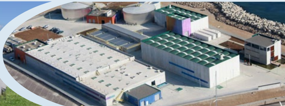
Algeciras WWTP, Spain BIOPUR®-DNK, BIOPUR®-NK and filtration Commissioning 2009, 204'000 p.e.
