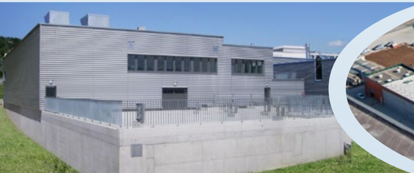
Meilen WWTP, Switzerland BIOPUR®-DN, BIOPUR®-NK and flocculation filtration Commissioning 2012, 52'500 p.e.
