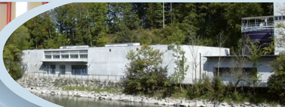
Worblental WWTP, Switzerland BIOPUR®-DN and BIOPUR®-NK Commissioning 2007, 140'000 p.e.
