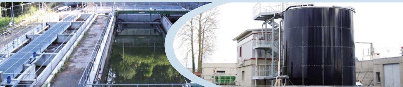
Jonschwil WWTP, Switzerland Commissioning 2004, 7'500 p.e.
