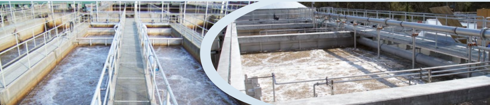
Chur WWTP, Switzerland Commissioning 2005-2007, 130'000 p.e.
