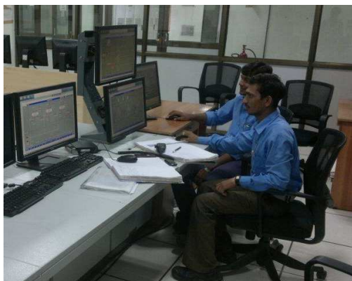
Figure 1 Essar Refinery - water reclamation plant control room
