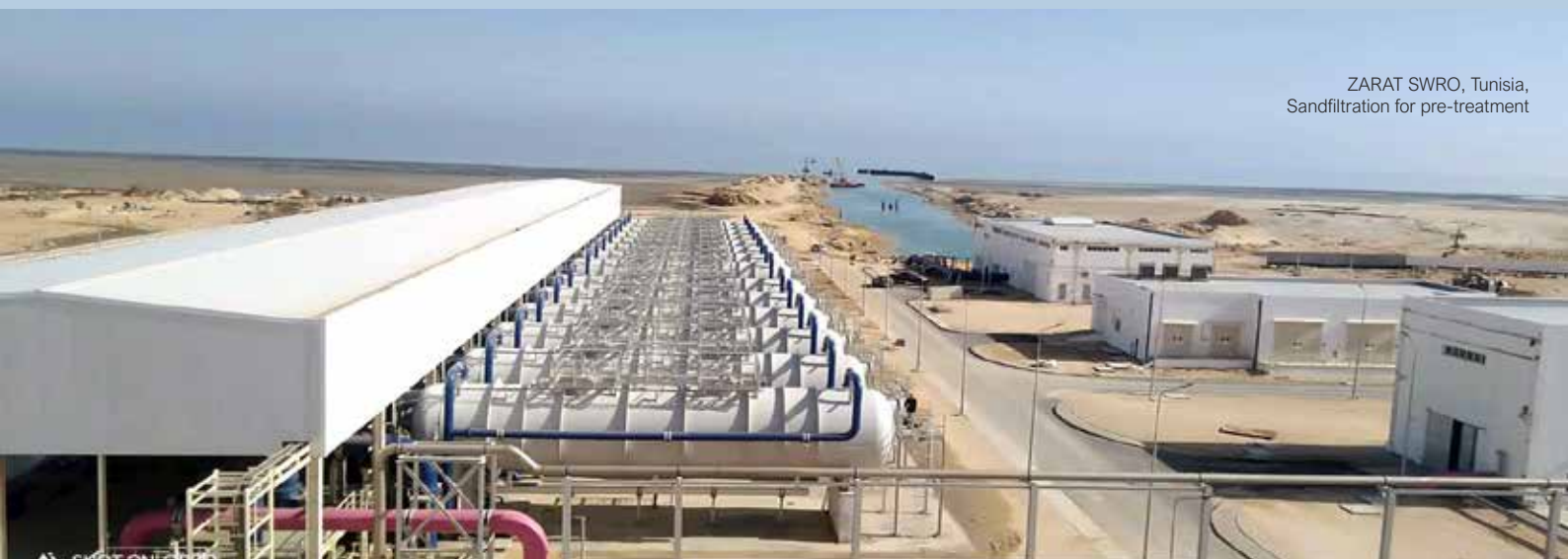
▲ ZARAT SWRO, Tunisia, 50,000 / 100,000 m 3 /d, RO system with Energy Recovery
