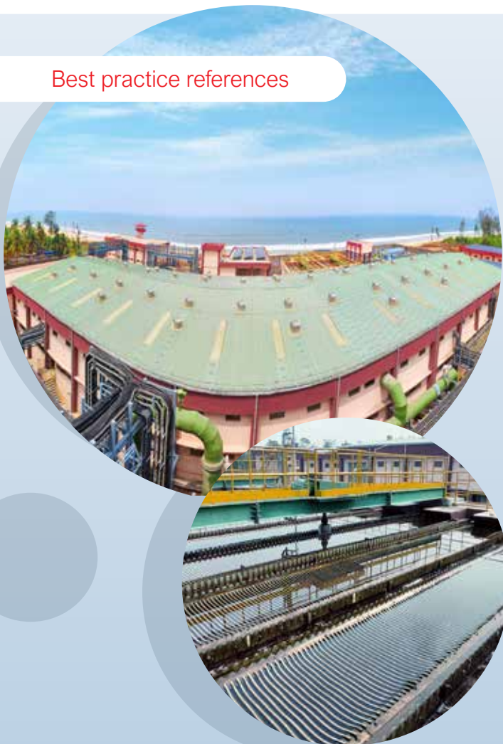
Lamella clarifiers – the WABAG OPUR-SK™ technology for highly effective pre-treatment
