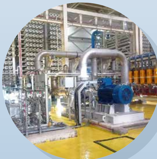
▲ ZARAT SWRO, Tunisia, 50,000 / 100,000 m 3 /d, RO system with Energy Recovery
