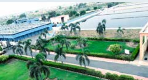
One City, One Operator: Wastewater Management for Agra and Ghaziabad, India, 2019-2029
