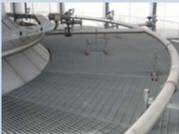
Homogenisation: gas injection
